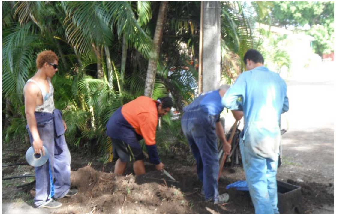
Installing water meter in Parekura
